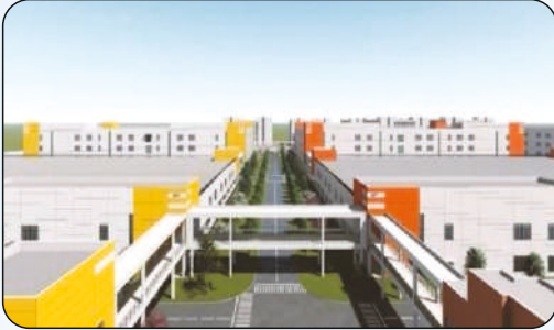
Project Name : FOXCONN Location : Hyderabad, Telangana
