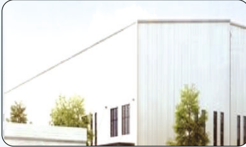
Project Name : ATL Battery Location : BAWAL, Haryana
